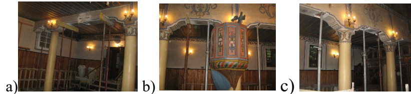
Fig. 1a, b, c. Replacing in certain places the longitudinal wooden beams located above the wooden columns with metal stands from the Hünebeck scaffolding on the A axis.
